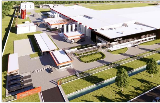
Coca-Cola Long An Greenfield LEED Gold Certificate
