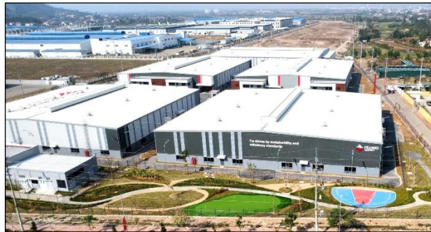
Frasers Property Dong Mai LEED Silver Certificate
