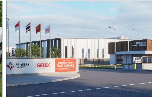
Frasers Property Yen Phong Expansion LEED Silver Certificate
