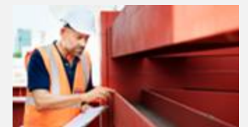
Paint Surface Inspection
